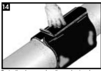
Centre the closure seal on the overlapping sleeve Using a gloved hand, press the closure seal firmly down onto the sleeve. Press from the centre to the ends to ensure good contact is made between the entire closure seal and sleeve.
