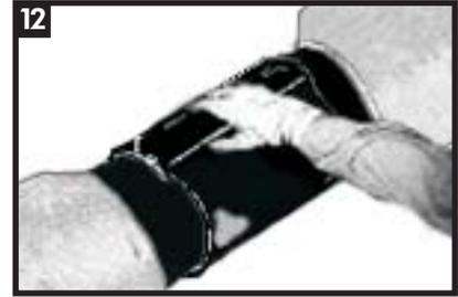
Press the closure firmly into place. Ensure the closure is in complete contact with the underlying sleeve.
