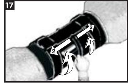
While the sleeve is still hot and soft, use a hand roller to gently roll the sleeve surface and push any trapped air up and out of the sleeve, as shown above. If necessary, reheat to roll out air.
