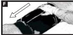
Gently heat the closure and pat it down with a gloved hand. Repeating this procedure, move from one side to the other. Smooth any wrinkles by gently working them outward from the centre of the closure with a gloved hand.
