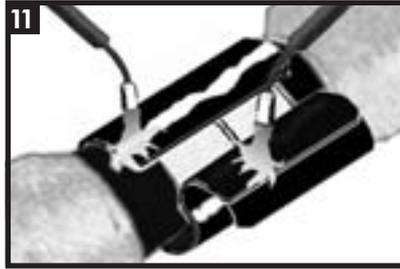
Gently heat the backing of the underlap, the adhesive side of the overlap and the adhesive side of the closure until it becomes shiny.
